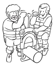
Cut the pipe square – the ends must **be square**. Guillotines are best. Remove the burrs if you've used a saw. Wipe the pipe inside 'n' out with a big towel first, then wipe the pipe using a handful of alcohol wipes (not just one). This cleans the pipe thoroughly! Remember the pipe must be dry and clean, clean, clean!! If you have lots of joints to do I suggest you buy a big container of
