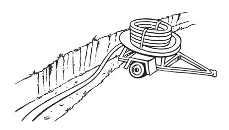
I've done a bit of pipe bursting in my time too, that's one of those in-line replacement trenchless technology methods where you have an ol' water main that you want to rehabilitate without using 'dig n lay' methods. I get lplex to make coils of 125mm PE pipe and get it made straight onto braked carousels like this......
