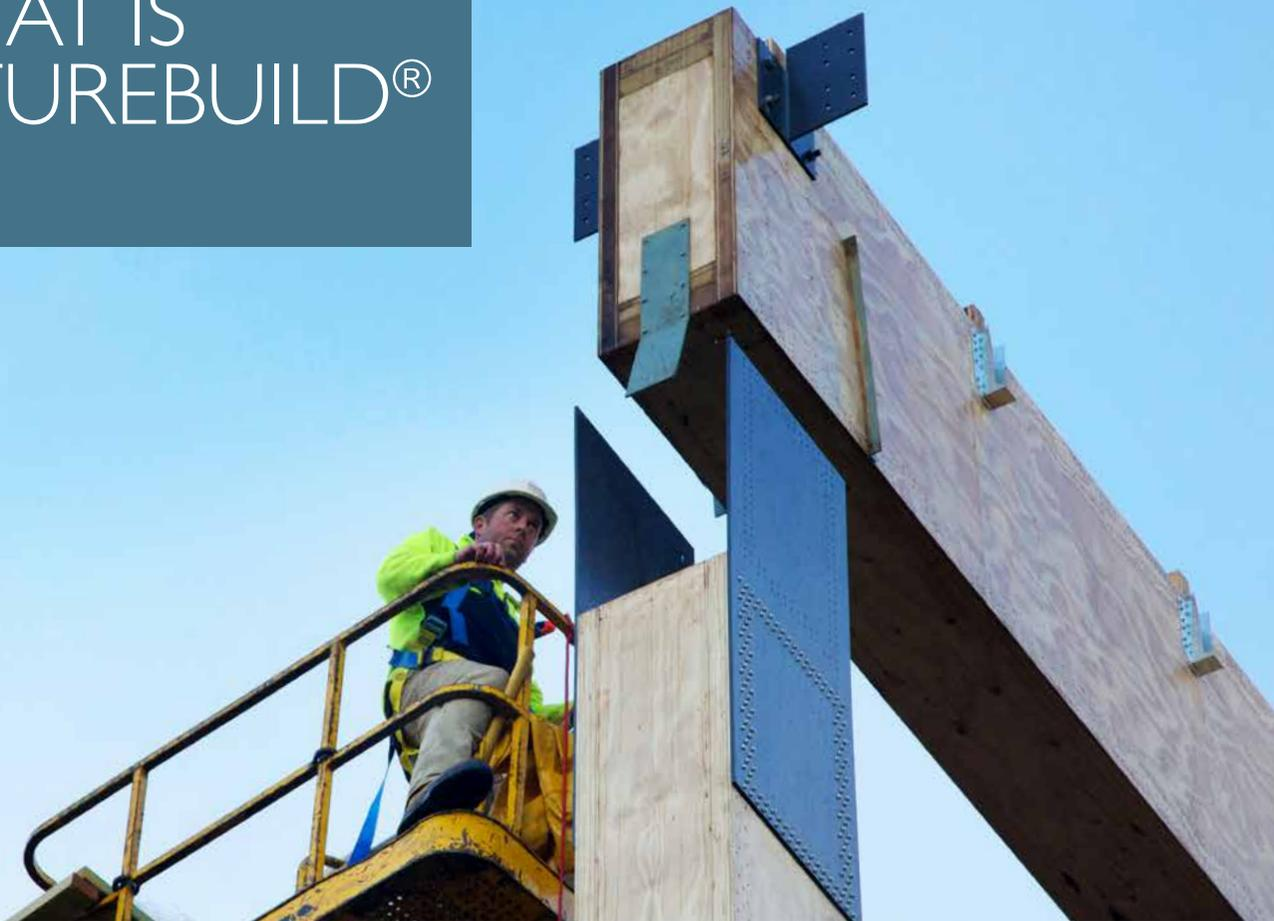
FUTUREBUILD® LVL (LAMINATED VENEER LUMBER) IS AN ENGINEERED WOOD PRODUCT THAT USES MULTIPLE LAYERS OF 3.5MM THICK WOOD VENEER LAMINATED TOGETHER UNDER PRECISE FACTORY CONDITIONS.
