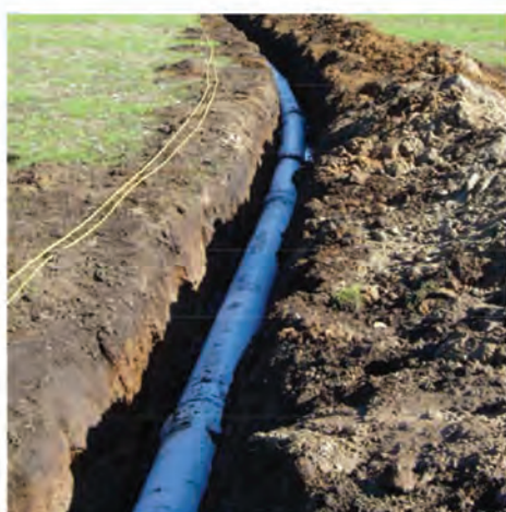
Figure 7.10: Curved pipeline installed ready for backfilling.
