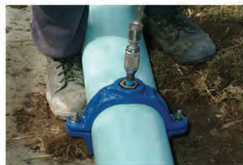
Figure 7.11: Taptite polymeric coated DI tapping band installed on an ApolloBLUE™ water main. Shown here is a brace and bit fitted with a hole saw being used for a "dry" tapping.
