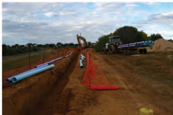
Figure 3.1: A combined trench installation using blue DN100 and purple DN150 ApolloBLUE™ for a dual water supply at Bamera, South Australia
