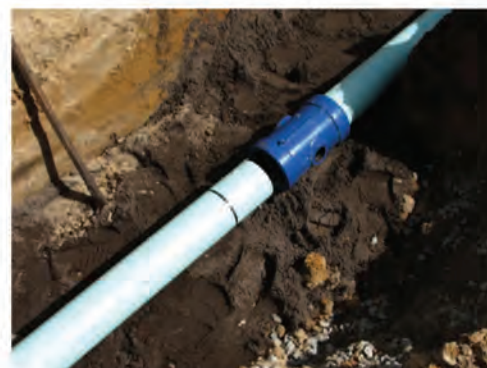
Figure 7.13: Tapped DI couplings can be used for service connections.
