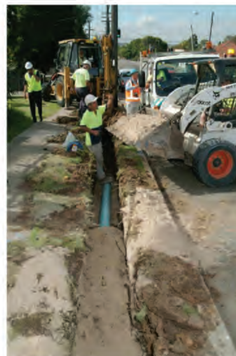
Figure 7.5: A granular embedment material should surround pipes and be adequately compacted in the side support zone before excavated material is placed into the trench.
