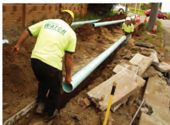
Figure 7.3: Faster installation is possible especially on congested sites owing to the pipes light-weight nature and minimal jointing force required when using ApolloBLUE™
