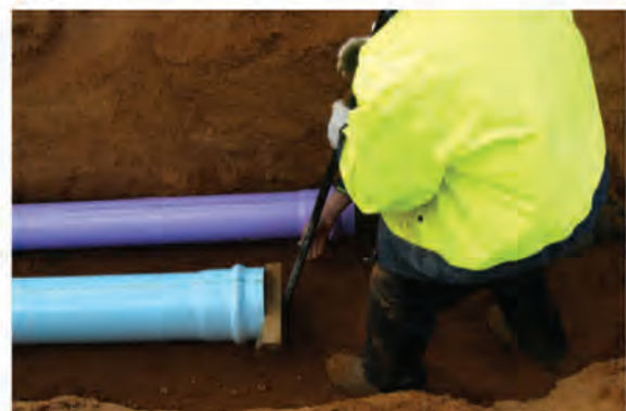
Figure 7.8: A DN150 ApolloBLUE™ pipe is being joined by pushing with a crow bar. Note: the pipe socket is protected from possible damage with a block of timber.
