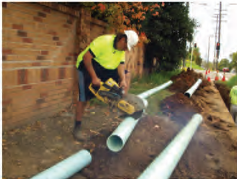
Figure 7.6: Powered disc cutter is being used to cut ApolloBLUE™ to length on site
