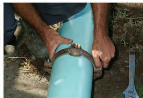
Figure 7.12: Most tapping bands providing full circle support to the pipe are suitable for ApolloBLUE™. A Milnes gunmetal band is shown here.
