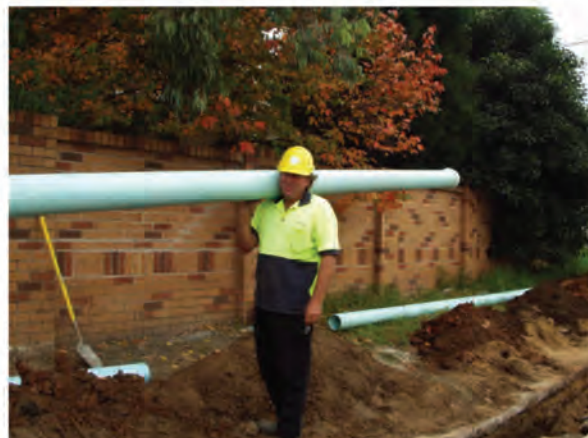
Figure 7.2: ApolloBLUE™ pipes are easily handled on site
