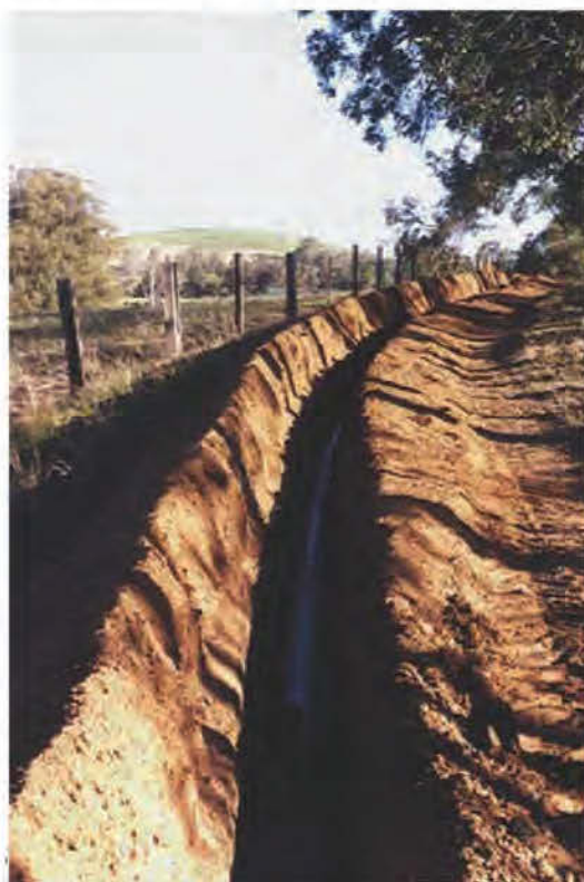
Figure 7.8 - DN 150 PN 6 S1 RHINO™ pipeline laid on a curved alignment near Broke, NSW
