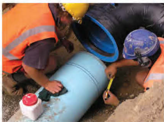
Figure 7.6 – New witness mark is being stencilled to cater for the ductile iron socket being used.
