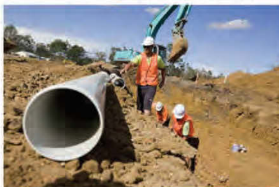
Figure 1.1 - WHITE RHINO™ PVC-M Pipes being installed at the Wimmera Mallee Pipeline Project, Victoria.
