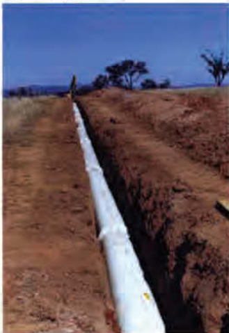
Figure 7.3 - DN450 PN 9 WHITE RHINO™ pressure pipe for irrigation supply in Hunter Valley, NSW
