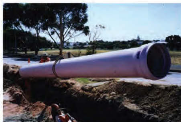
Figure 3.1 - Iplex DN450 PN12 Series 2 PVC-M purple pipes for recycled water at Willunga, South Australia.
