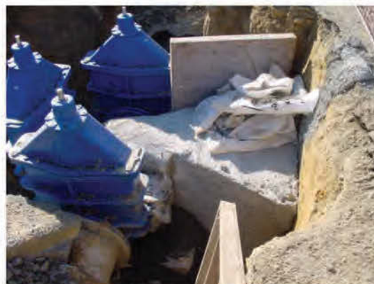
Figure 6.2 - Concrete thrust block, correctly oriented to transfer the hydraulic thrust to the specially trimmed undisturbed soil of the vertical
