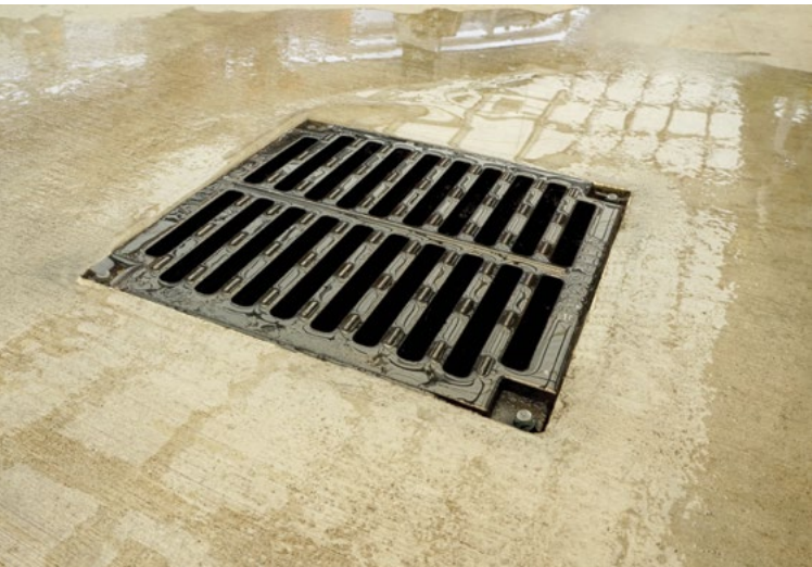
Polymer Concrete Pits
