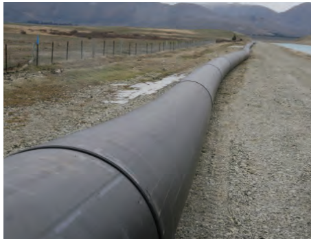
Tekapo diversion main
