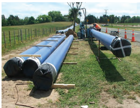
Papamoa trunk water main
