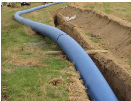
Aokautere falling water main
