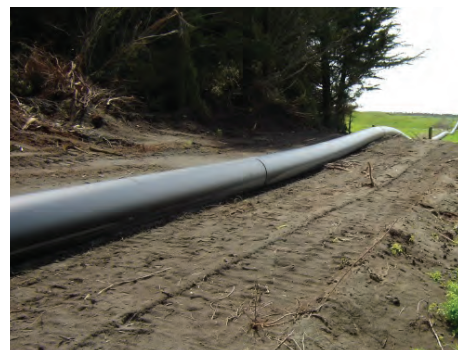
Waitara to New Plymouth wastewater rising main
