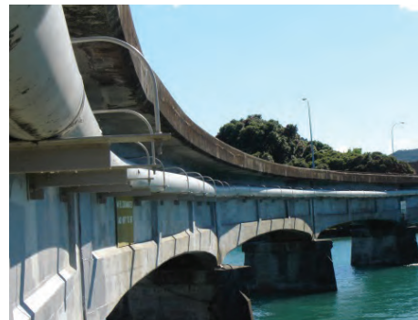
Gisborne wastewater rising main
