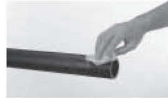
3 Clean pipe(s) in fusion zone with PE cleaner (Tangit or equivalent)
