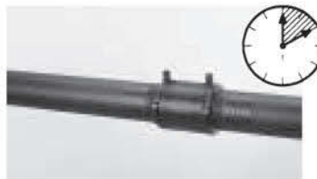
16 Wait maximum cooling time before pressure test
