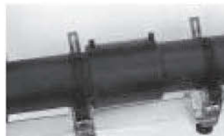
10 Firmly fasten integrated clamps
