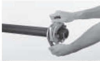
2 Remove (scrape or peel) oxide film of pipe(s) using correct tooling
