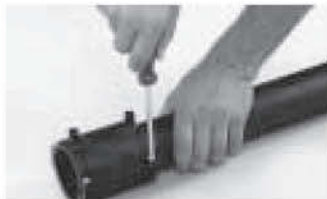
7 Firmly fasten integrated bracket
