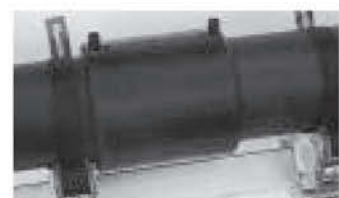
13 After fusion completed check machine display for error message then visually check all parts of the fitting and fusion indicators
