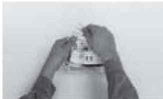
5 Remove fitting(s) from the packaging without touching the fusion surface, wipe surfaces with cleaner
