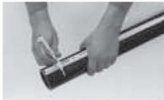
4 Mark the insertion depth on the pipe
