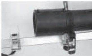
8 Mount and fix assembly clamps
