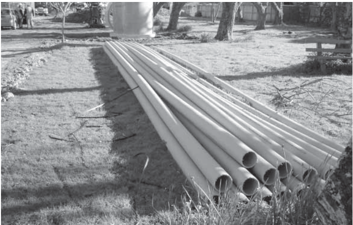
POLIDRAIN 17 ready to be welded for installation.
