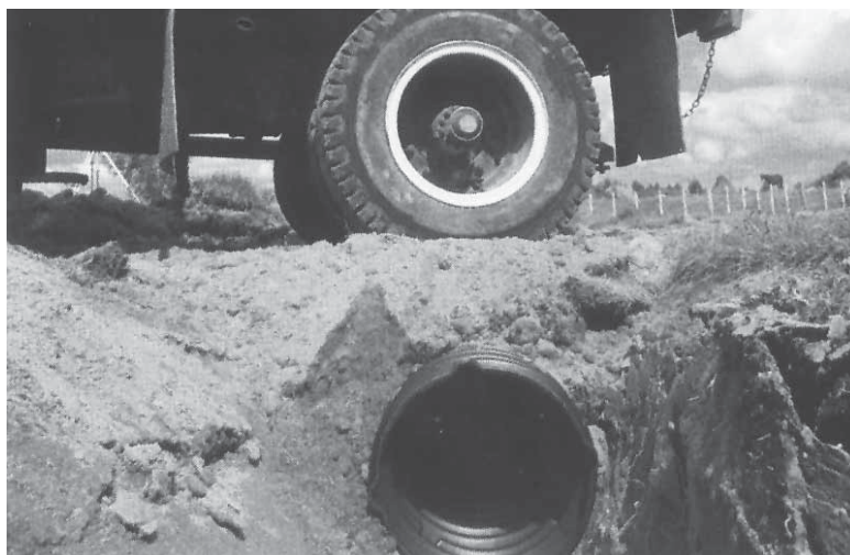
DN600 Laylite Culvert Pipe under a construction site access road
