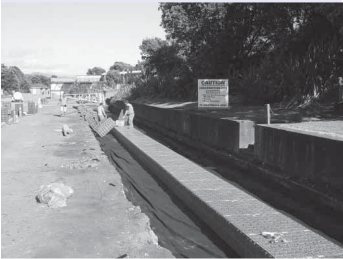
Aquacell shallow conveyance and infiltration gallery under construction.
