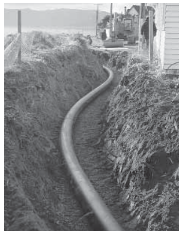
DN315 PN 16 PE100 watermain with butt fusion joints.
