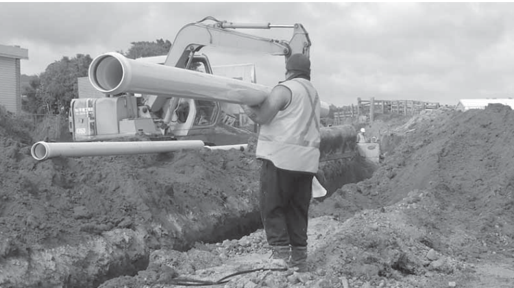
Manual site handling of light weight DN 150 S2 PN 16 APOLLOBLUE
