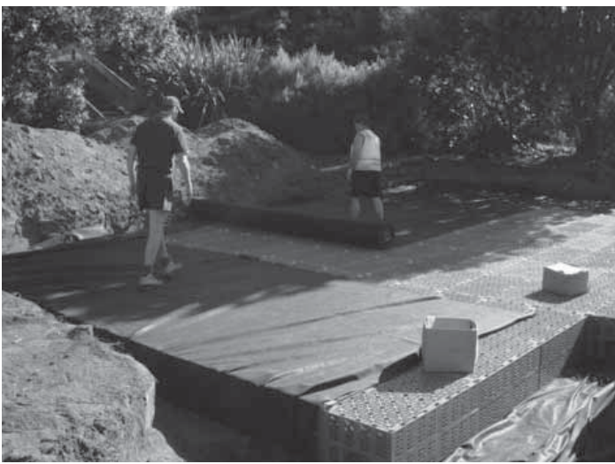
Wrapping an Aquacell infiltration gallery in geotextile fabric prior to backfilling.
