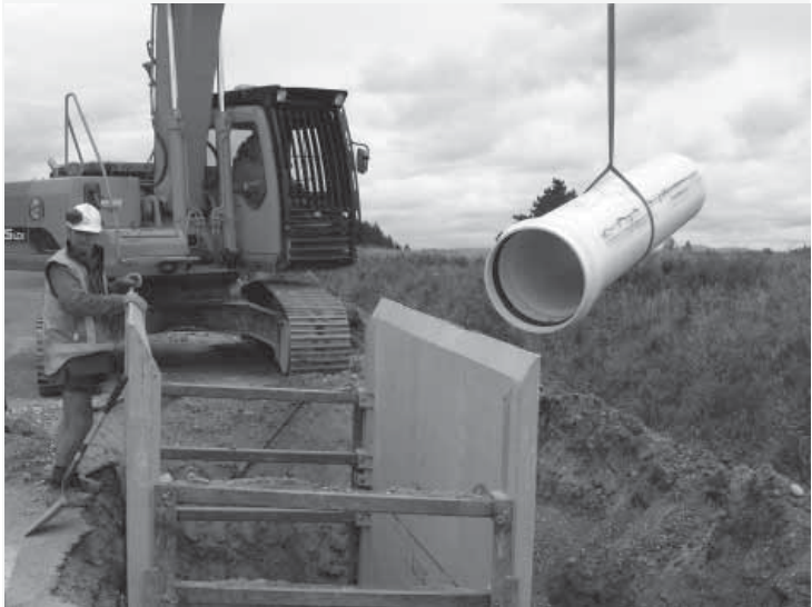
Installation of 3 metre lengths 575 PN6 PVC-U pipe in trench shields as part of a storm water discharge line.
