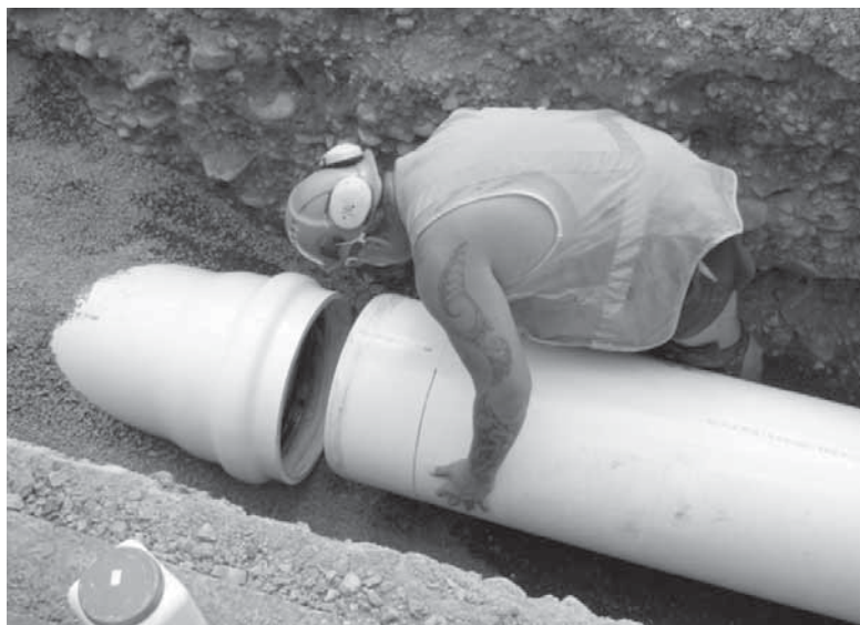
Joint assembly on NOVAKEY DN 450 PN12 watermain under a sealed main highway.
