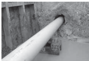
Assembly and installation of DN150 RESTRAIN gravity sewer, replacing an old EW sewer by pipe reaming with a horizontal directional drill.
