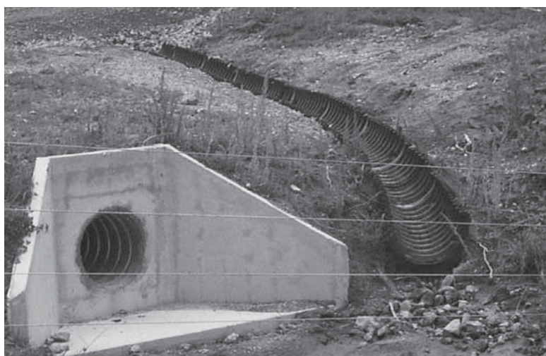
DN 400 Laylite Flume installation showing required anchor attachments
