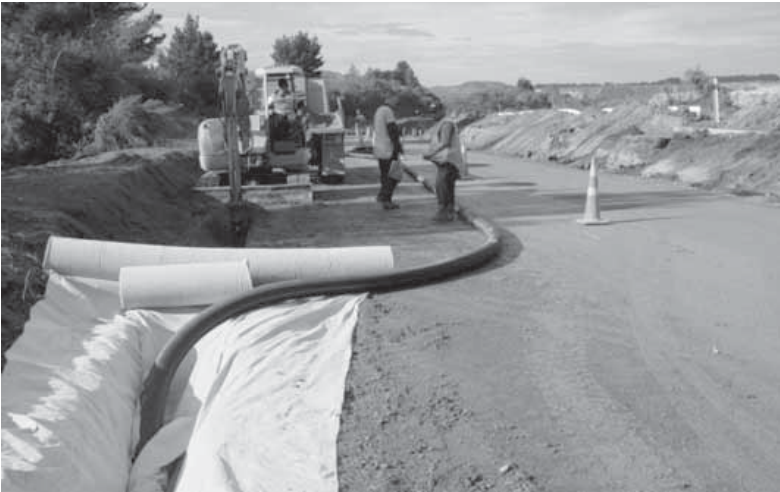
NEXUS HI-WAY interceptor drain installation, with Geotextile filter / aggregate filter surround system under main sealed road
