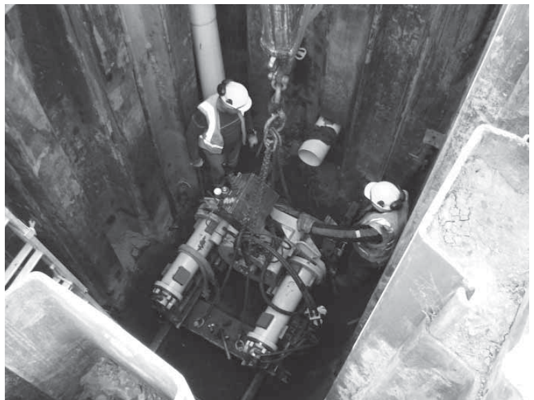
Microtunnelling installation of DN 225 (250mm OD) RESTRAIN
