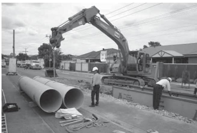
DN750 GRP waste water line being prepared for installation.
