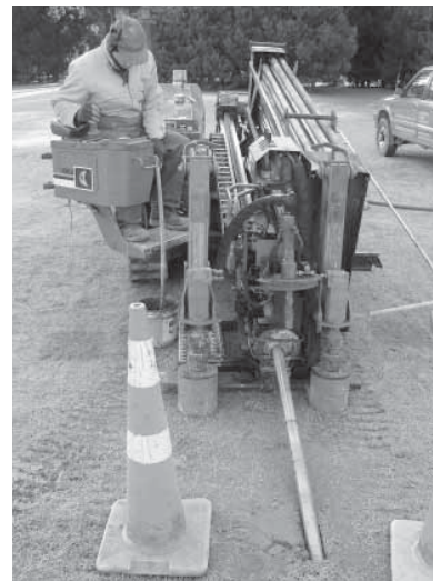
Assembly and installation of DN150 RESTRAIN gravity sewer, replacing an old EW sewer by pipe reaming with a horizontal directional drill.
