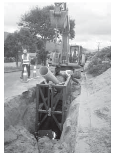
Installation of DN300 BLUE BRUTE PN12 watermain under main sealed road.
