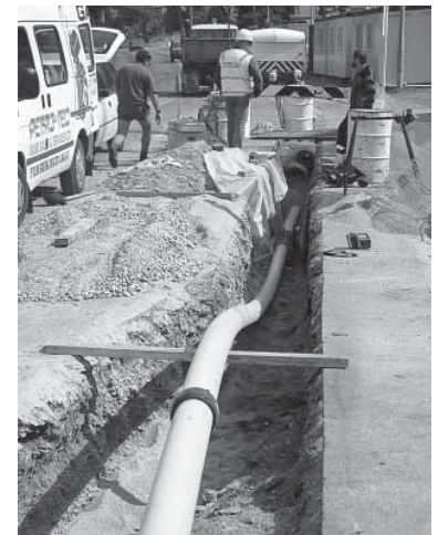
DN110 PE 80 Gas Pipe with electro fusion joints.
