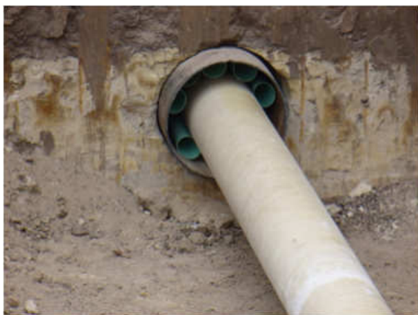
Figure 6.5 – DN250 SN10000 FLOWTITE™ being inserted into a host pipe. The allowable grouting pressure can be obtained from Table 6.7
