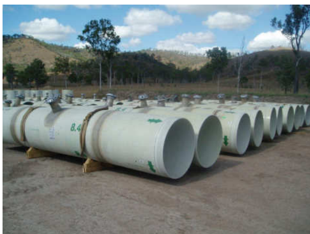
Figure 7.11 – Flanged off-takes for scours – Note the stub flanges and backing plates, which are the preferred option
