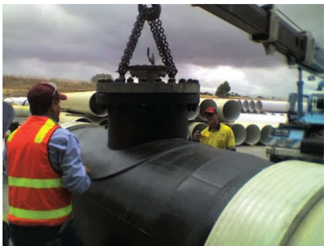
Figure 3.3 – DN1200 x 600 Flanged Access and Air Valve tee assembly with spigot inserted into DN1200 PN25 FLOWTITE™ coupling
