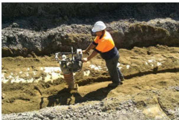
Figure 6.4 – Compacting sand embedment material in the side support zone of a DN1000 FLOWTITE™ pressure pipeline
