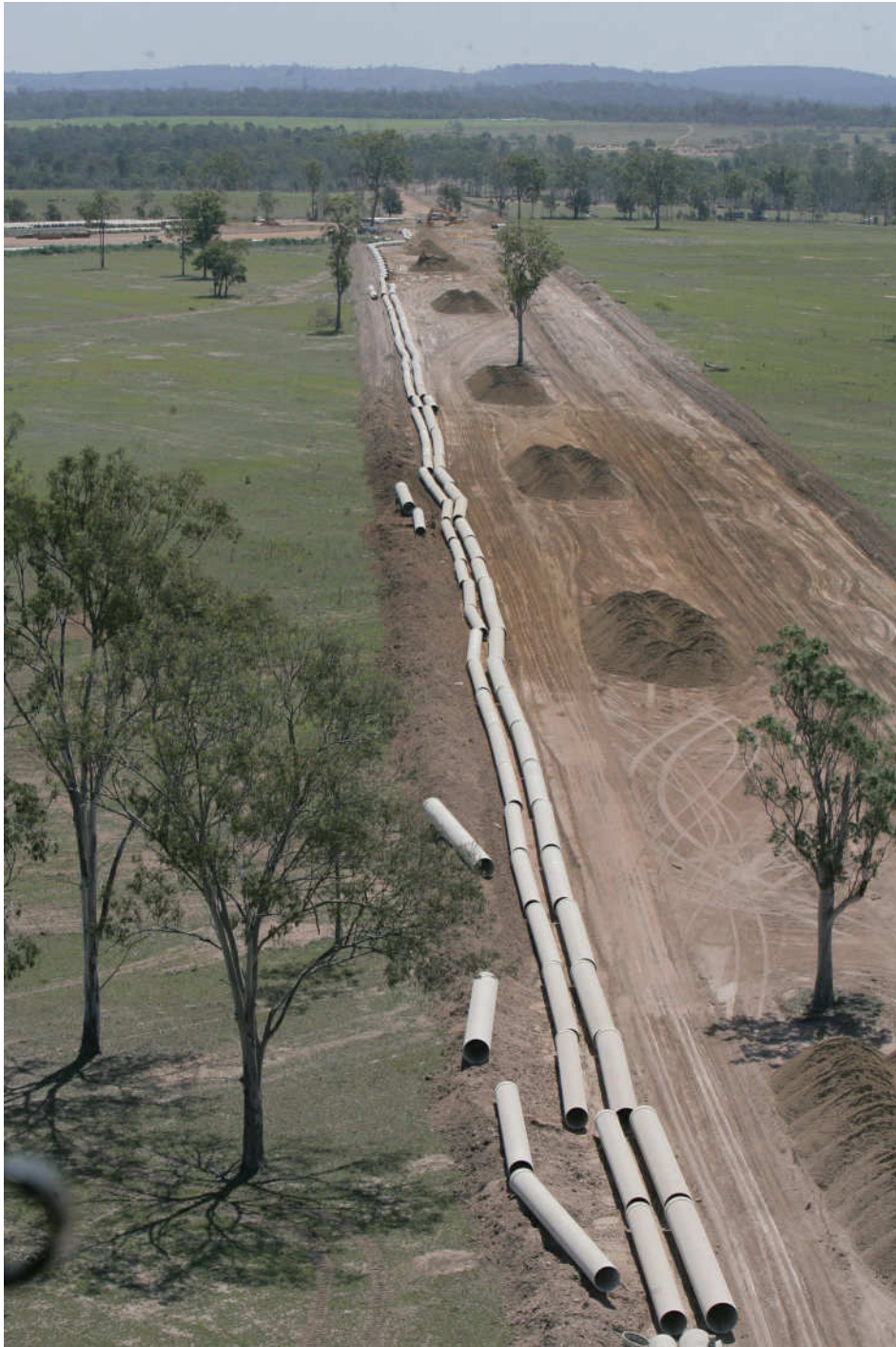
Figure 1.5 – DN1000 PN16 FLOWTITE™ pressure pipes and GRP fittings for a 63km recycled water supply line for the Lowood to Caboonbah pipe section, Western Corridor Queensland
