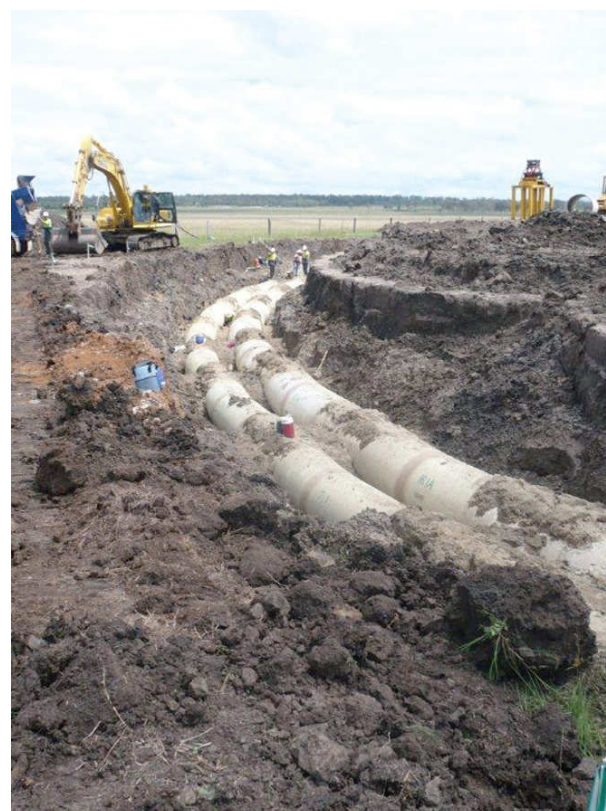
Figure 7.8 – FLOWTITE™ GRP pipes designed for curvilinear alignment and angular joint deflection
