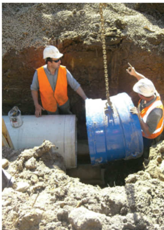
Figure 3.1 – Examples of polymeric coated ductile iron fittings with Griptite® seals suitable for use with FLOWTITE™
