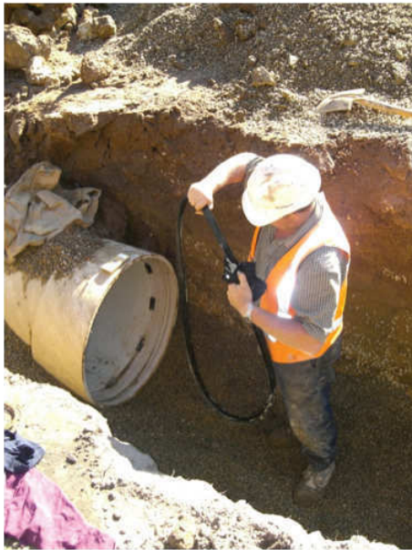
Figure 7.4 – Inspecting and cleaning the coupling grooves and ring before joining DN750 FLOWTITE™ pressure pipes
