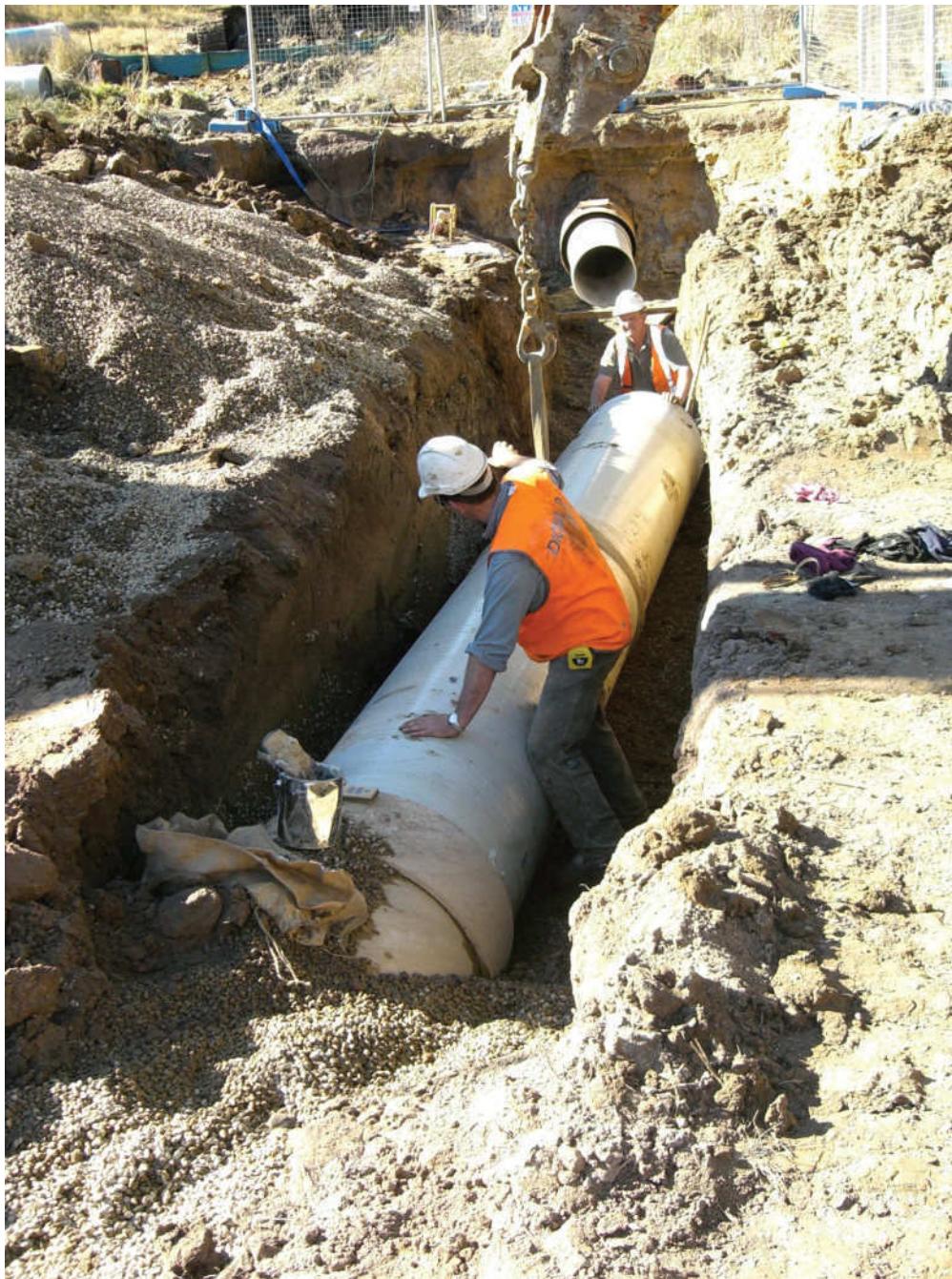
Figure 2.3 – DN750 PN16 FLOWTITE™ water supply line for the City of Wyong NSW
