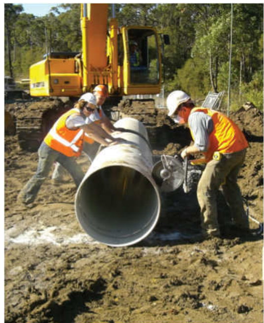
Figure 7.6 – A petrol powered disk cutter is used to cut the pipe
