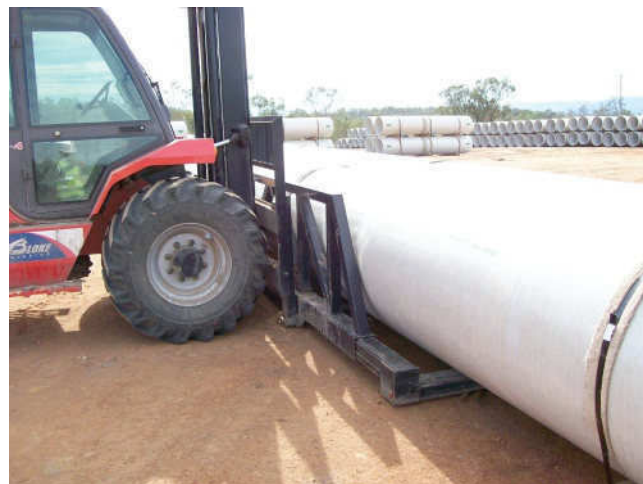
Figure 6.13 – FLOWTITE™ pipes in 12m lengths, being unloaded on site with a suitable forklift, load rated to suit lifting requirements
