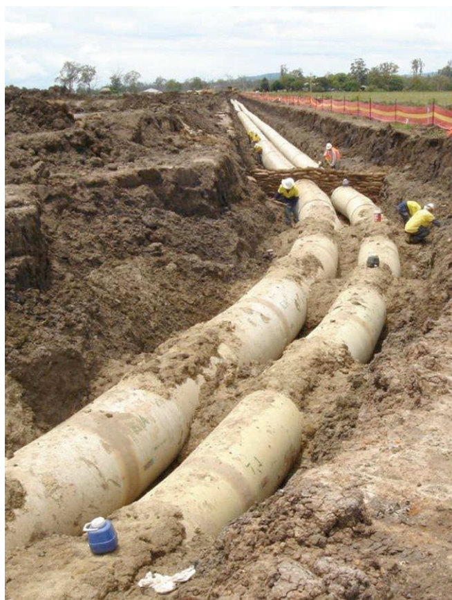
Figure 2.2 – DN1000 PN16 SN10000 FLOWTITE™ pressure pipes with special long length 'angled' GRP bends designed for 'curvi linear alignment' and installed at Wivenhoe Dam in South East Queensland
