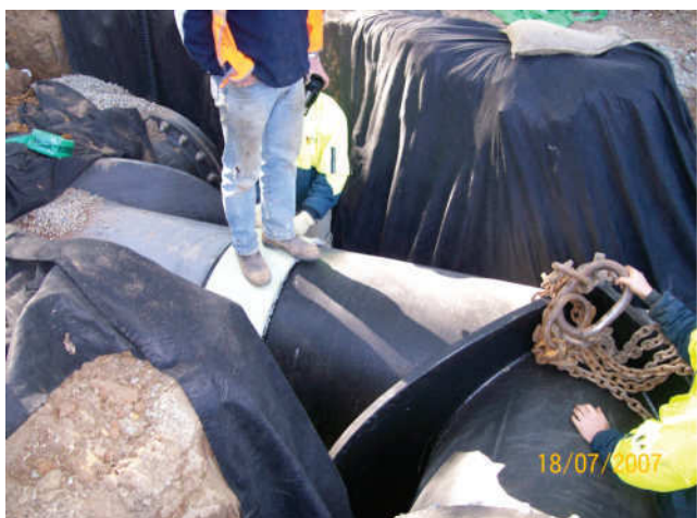
Figure 3.2 – DN1000 spigot epoxy coated steel fitting joined to a PN16 SN10000 FLOWTITE™ water main using a FLOWTITE™ GRP coupling
