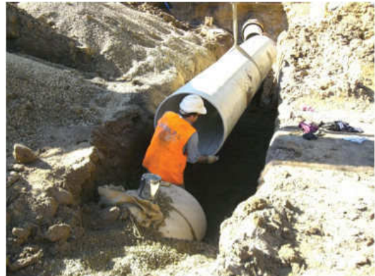
Figure 7.5 – Applying an approved jointing fluid to the pipe spigot prior to inserting the spigot into the coupling
