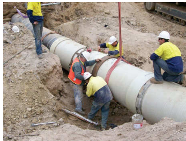
Figure 7.14 – DN10000 FLOWTITE™ GRP adjustment pipe being inserted as a "closure pipe" using FLOWTITE™ couplings for slip action
