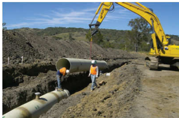
Figure 6.9 – DN1000 PN16 SN10000 FLOWTITE™ pressure pipes being installed on a major recycled water pipeline near Wivenhoe Dam in South East Queensland
