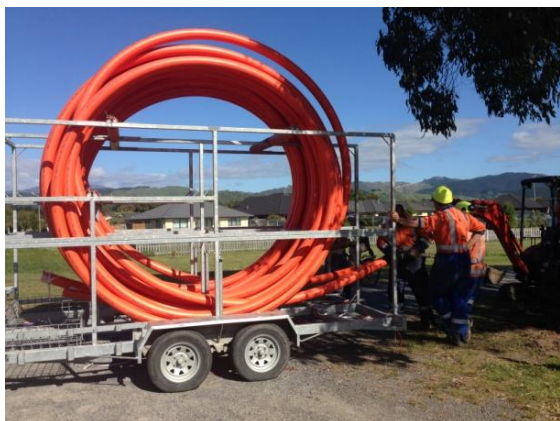
Two DN 110 PE electrical ducts in 50m coils on a dual-coil dispensing trailer
