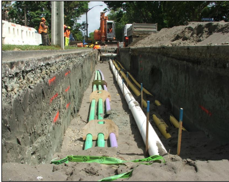
100 mm green PVC Telecommunication ducts, showing horizontal separation in the trench space from other services such as recycled water (purple), potable water (white) and gas (Yellow) Also trench wall is marked to locate backfill compaction zones above the pipes
