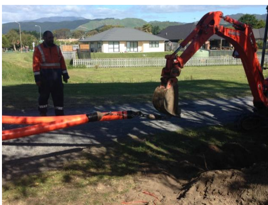
DN 110 PE electrical ducts with pull heads in place, ready for pull-in by horizontal directional drilling
