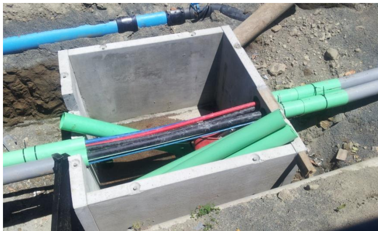
DN 32 PE sub- ducts inside 100mm PVC carrier ducts, at a roadside connection pit
