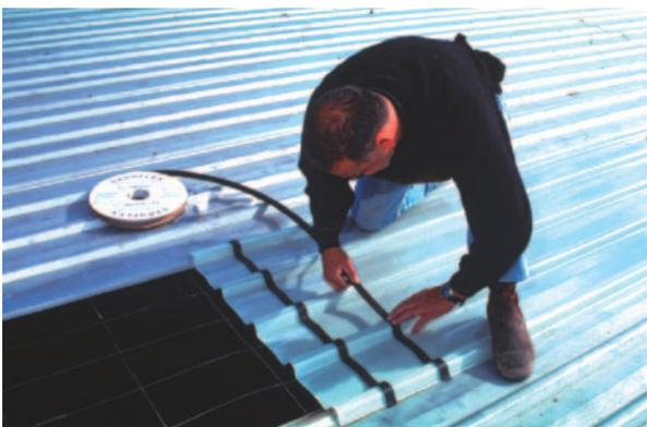
Furthermore, gaps in the pans of dissimilar materials can occur. The foam tapes fill up these spaces much more effectively than silicone. The end lap fixing methods are the same for metal onto fibreglass, fibreglass onto fibreglass, or fibreglass onto metal.
